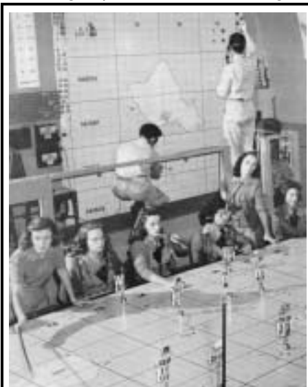
Women's Air Raid Defense (WARD) staffers on the job at a information and control center in 1943 or 1944. Behind is the radar plotting board, which displays data received from radar stations around the island. Workers positioned markers on the large "shuffleboard" at the center of the room to keep track of contacts.
