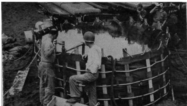
IWO WATER works was set up while the battle still blazed. Steaming hot water comes from distillation unit to reservoir.
